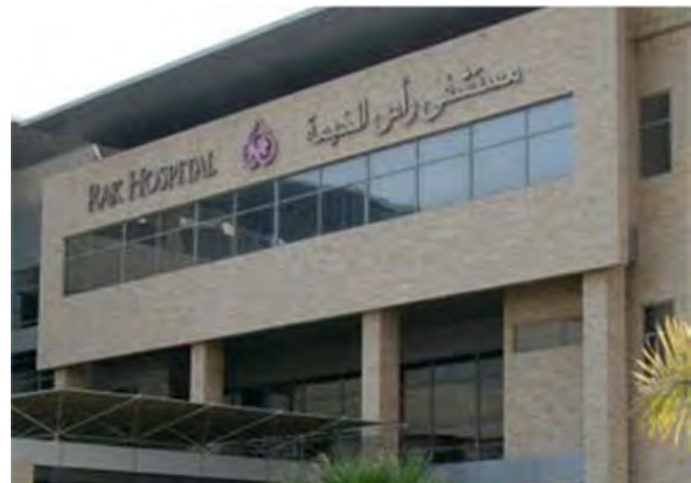
Ras Al Khaimah Hospital
